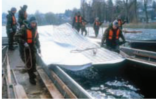
⌘ p. 296 Fig. 4.29 In 1998/99 geotextile with reinforcement lattice was installed and covered with a layer of gravel in Ermatingen-West (CH-TG-02).
