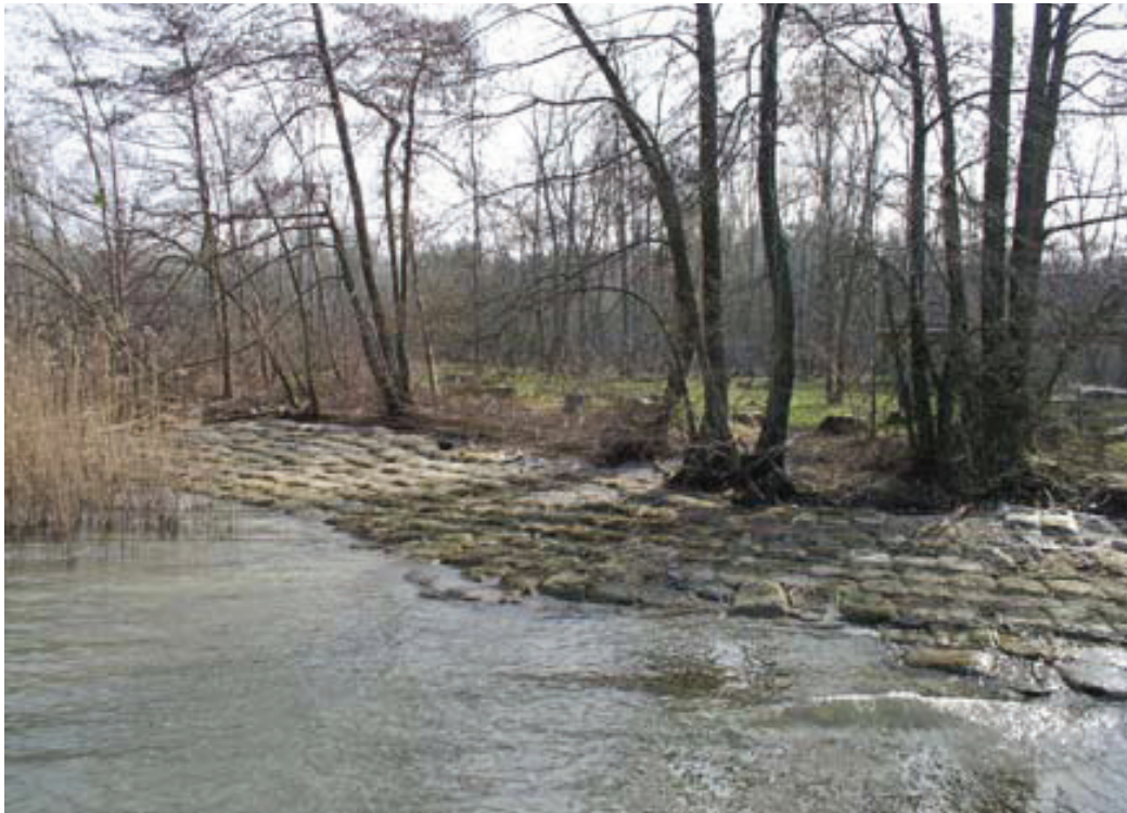
⌘ p. 296 Fig. 4.32 Protection measures (gravel in geotextile bags) were put in place in the submerged areas of the site Vernay–En Chéseau (CH-FR-08) in 1992.
