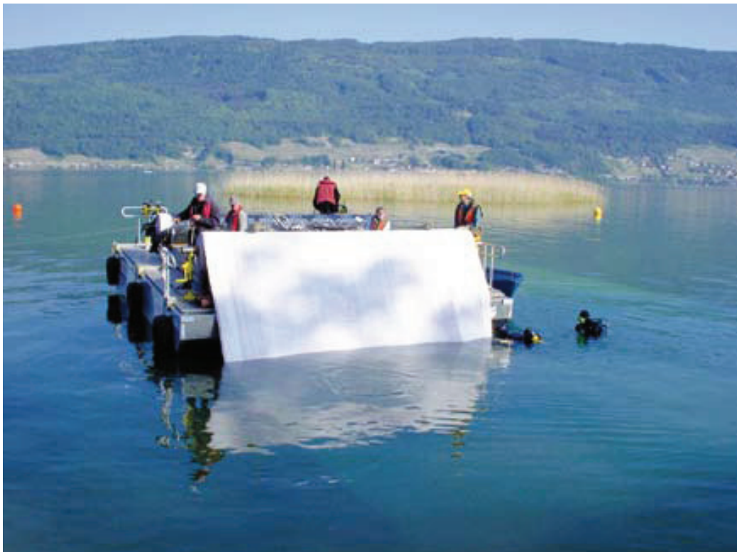
κ p. 295 Fig. 4.28 The Archaeological Service of canton Berne (Switzerland) has developed a special floating device for covering the well-preserved settlement layers with geotextile and gravel.
